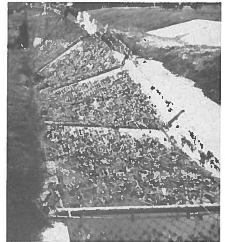
Fences in floodways often catch leaves and other debris that obstruct flood flows. Break-away fence posts, an example of projects eligible under the HMGP, allow floodwaters to pass safely downstream.
