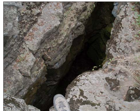
A 65-foot-deep sinkhole near Honey Creek
