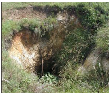
Sinkhole near Mill Creek
